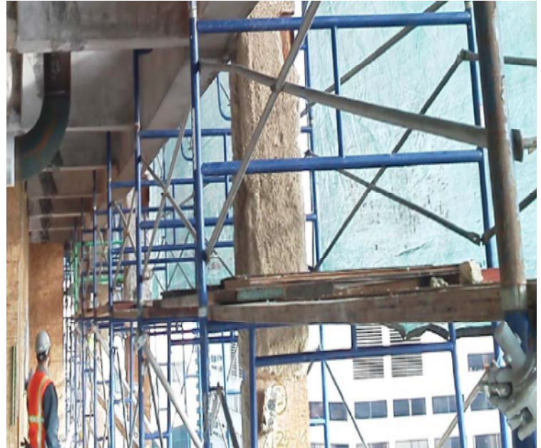
Penthouse Level 18 perimeter scaffolding
