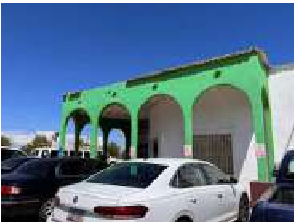
Façade facing parking lot
