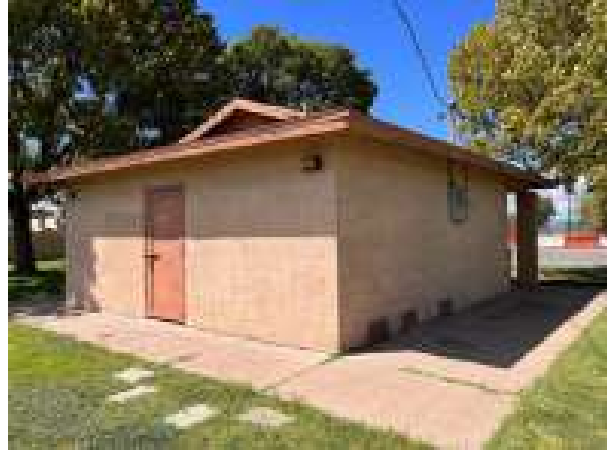
Rear and northern façade
