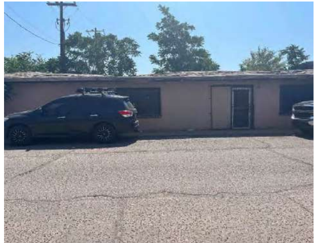
Building 1, Customs Avenue
