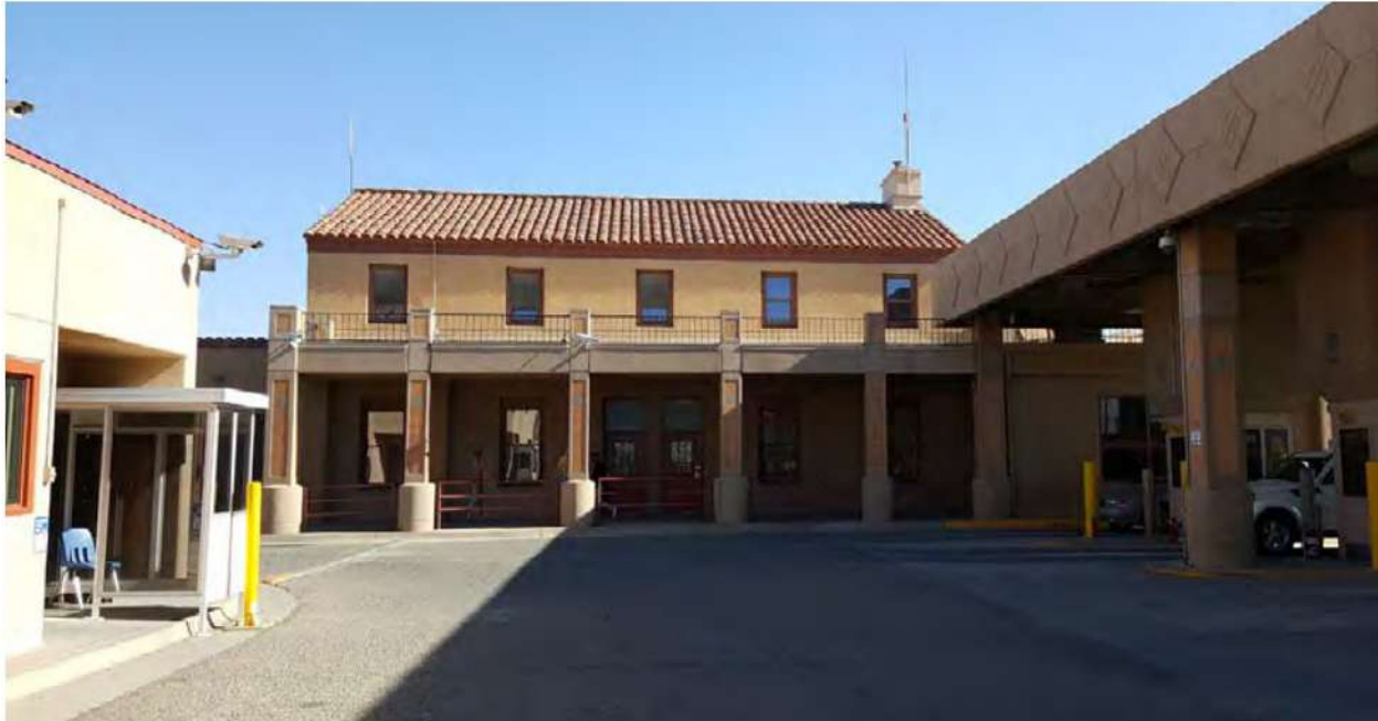
Figure 1-5. Historic Main Building – Facade
