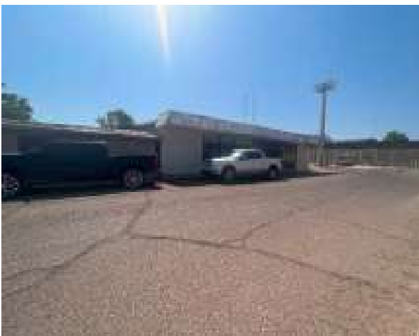
Building 2, Customs Avenue
