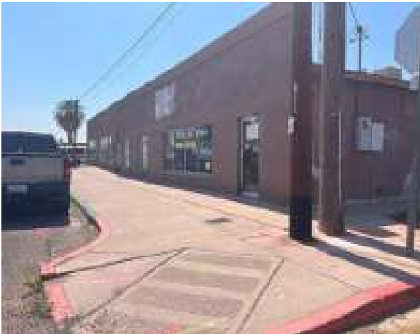
Commercial Building, 201 E. 1st Street
