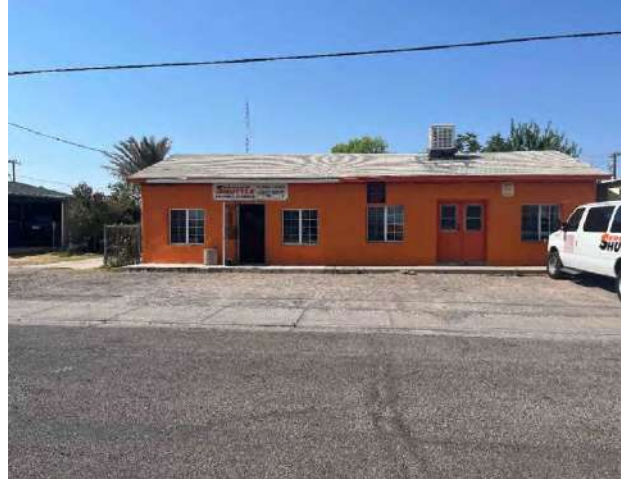
Commercial Building, 231 E. 1st Street
