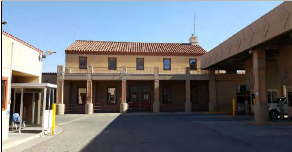
Figure 5. Historic Main Building – West Facade
