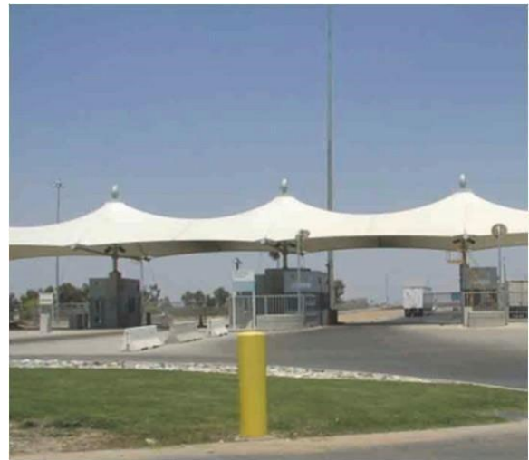
Illustration 19: Primary Inspection Canopy comprised of steel. It is measured and assigned because it covers an inspection-related function.
