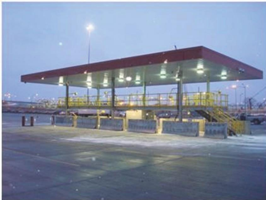
Inspection Catwalk with Canopy
