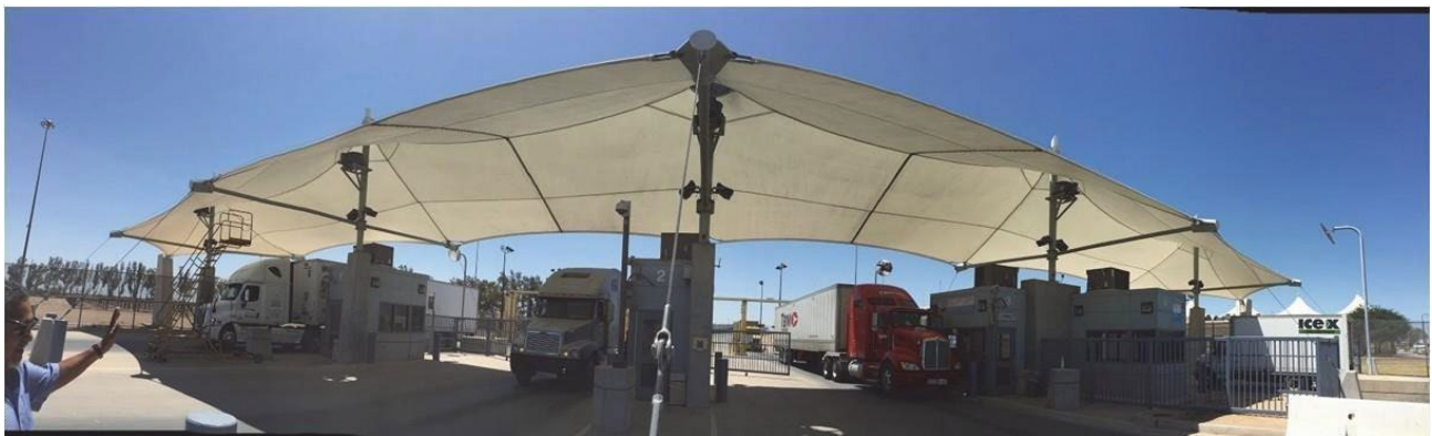
Commercial Primary Inspection
