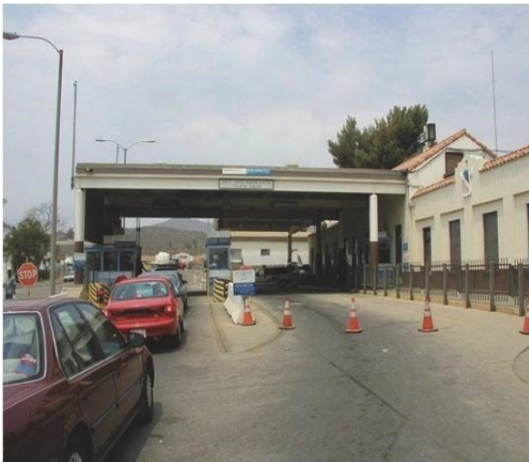
Illustration 18: Primary Inspection Canopy that also covers an area used for processing pedestrian traffic (on right side of picture). The pedestrian processing area is included in the primary canopy square footage.
