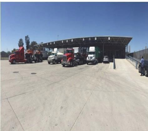
Commercial Outbound Inspection - Export Building
