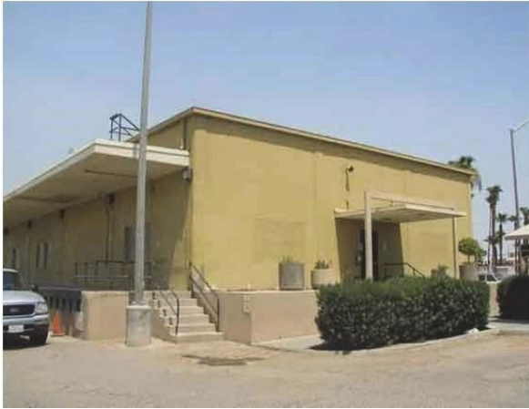
Illustration 16: Commercial Inspection Building. This building has two canopies. A commercial secondary inspection dock (left) is measured and assigned. The canopy on the right serves no inspection-related function and is not measured or assigned.
