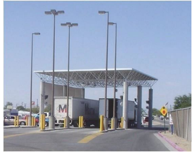
Illustration 13: Commercial primary inspection area with canopy and no inspection booth. The canopy is considered real property and there is an inspection-related activity being performed, so it is measured and assigned.
