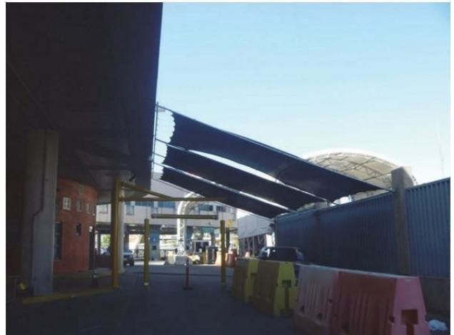
Illustration 11: The temporary canvas that is connected between the two buildings is not measured or assigned.
