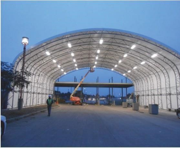
Illustration 12: Outbound inspection canopy is considered real property and is measured and assigned.
