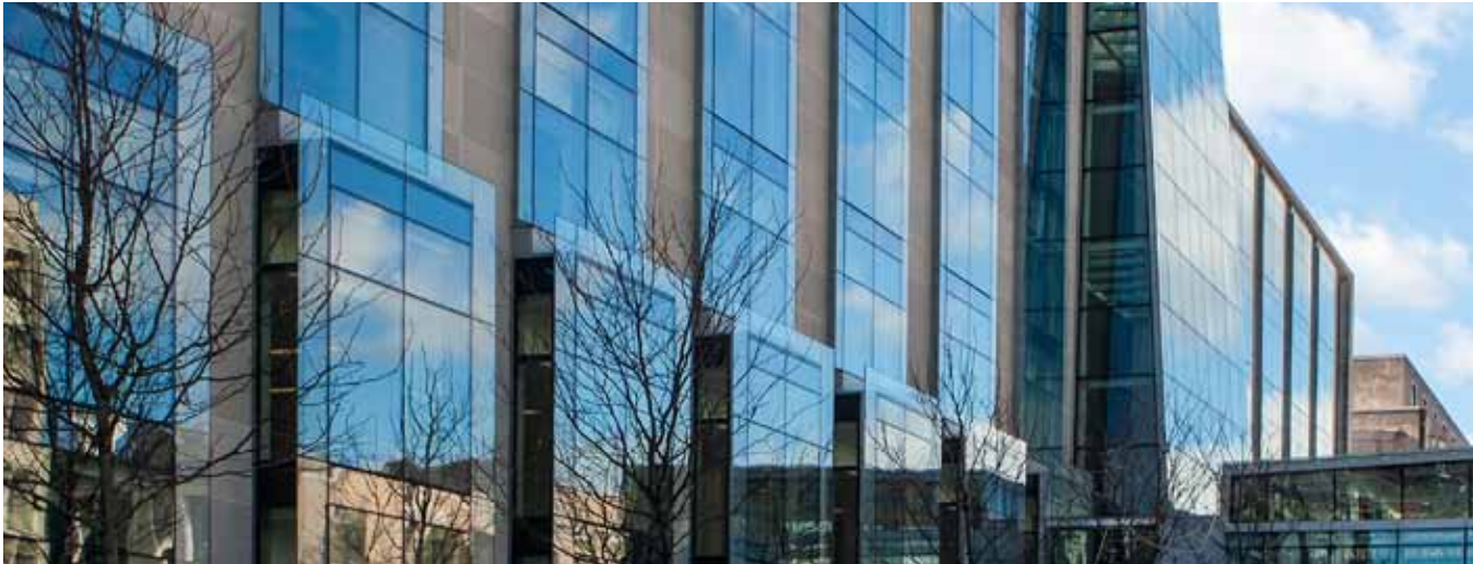
Federal Office Building 8, Washington, DC
