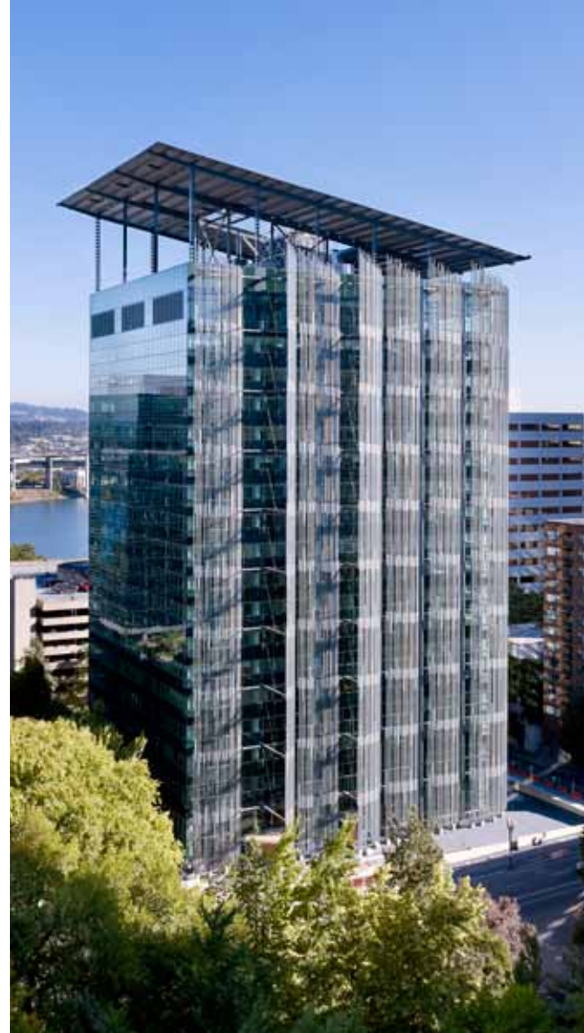
Edith Green - Wendell Wyatt Federal Building, Portland, OR
