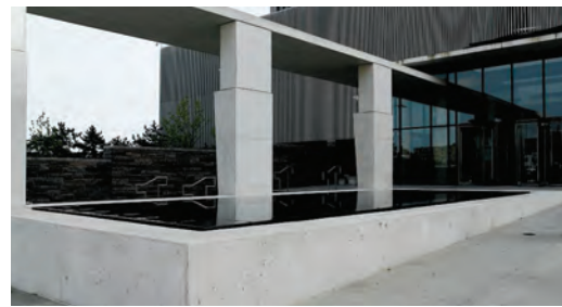
Richard Bolling Federal Building, Kansas City, MO
