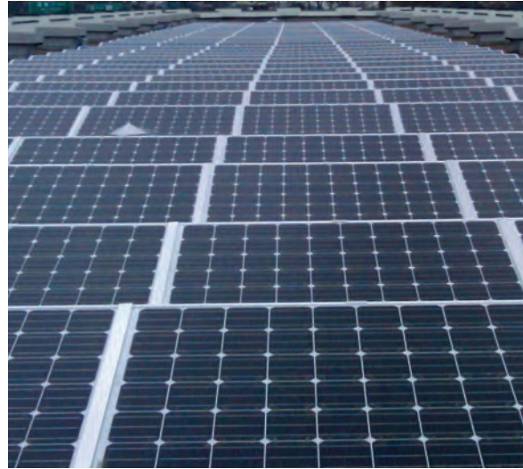
Juarez and Lincoln Land Port of Entry, Laredo, TX
