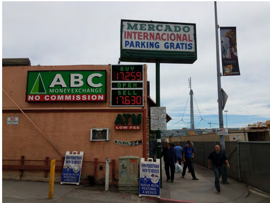
Photograph 1: View of the northwestern portion of the site (747 E. San Ysidro Boulevard).
