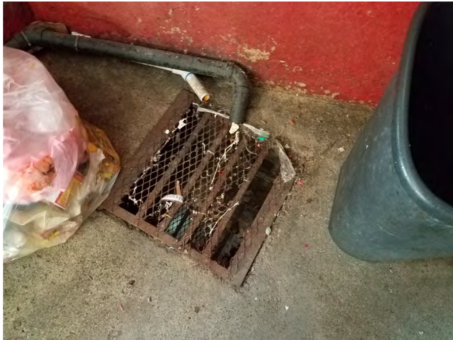
Photograph 16: View of storm drain near the fruit stand area.
