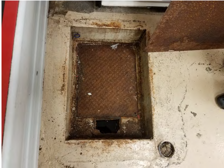
Photograph 13: View of grease interceptor access panel, located at the meat department of the Mercado International 88 suite (747 E. San Ysidro Boulevard).
