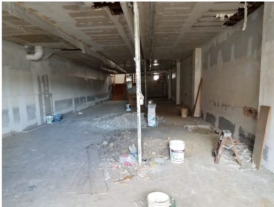
Photograph 4: View within the vacant suite of 751 E. San Ysidro Boulevard building.
