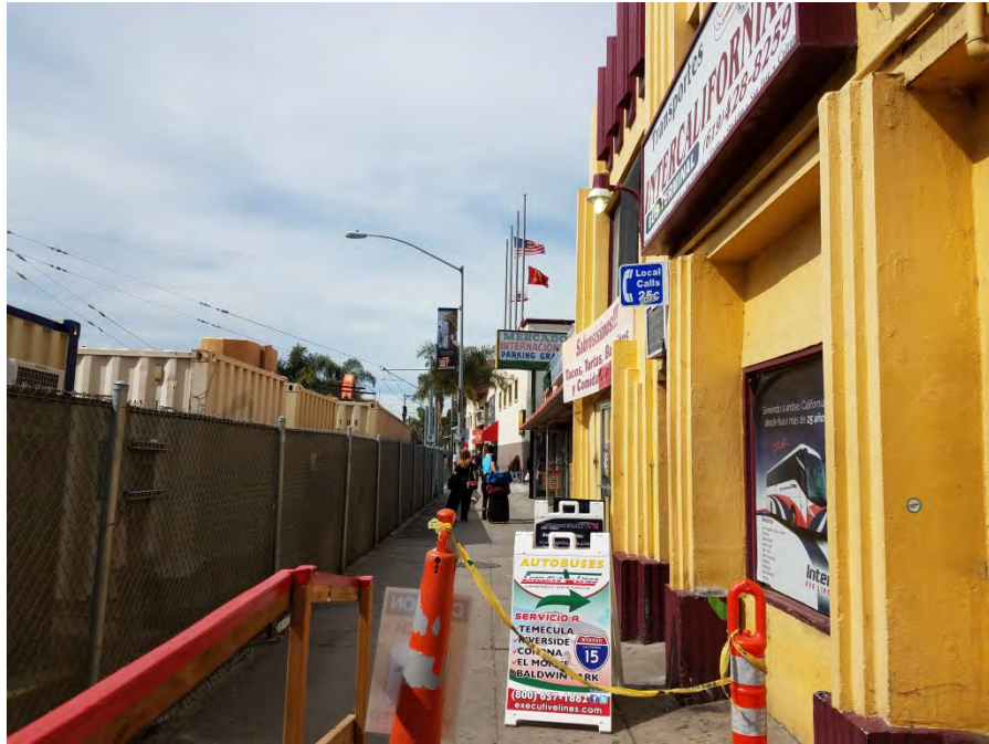
Photograph 3: View of the 751 E. San Ysidro site building, facing north-northwest.
