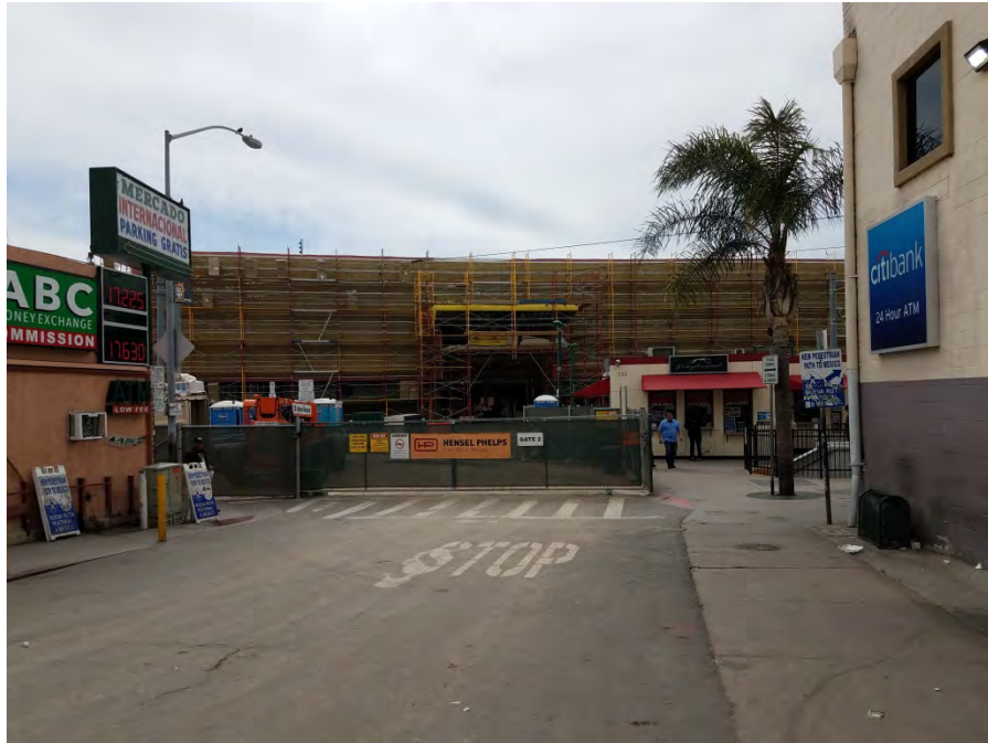
Photograph 23: View along Rail Court, facing southwest.
