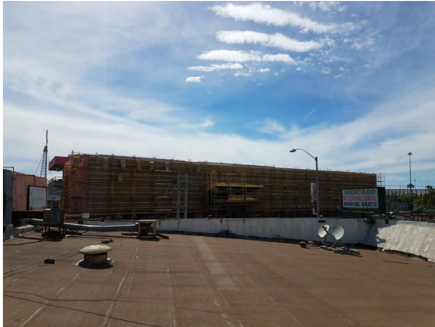
Photograph 17: Roof view of the 747 E. San Ysidro Boulevard building, facing west.
