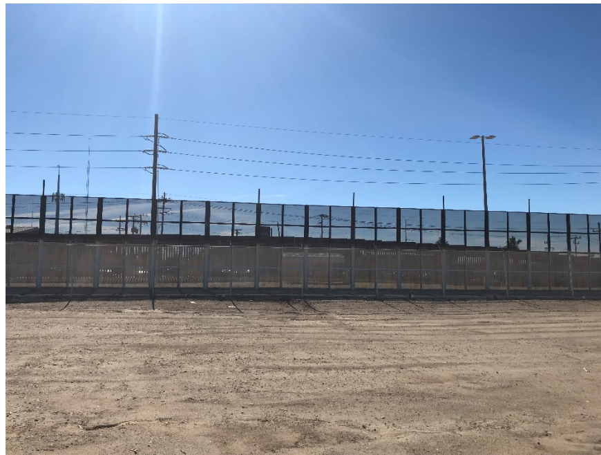
Figure 3-5. View of Pedestrian Fence Located South of the San Luis I LPOE
