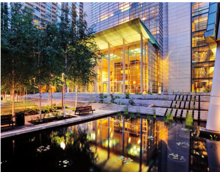
US District Courthouse - Seattle, WA
