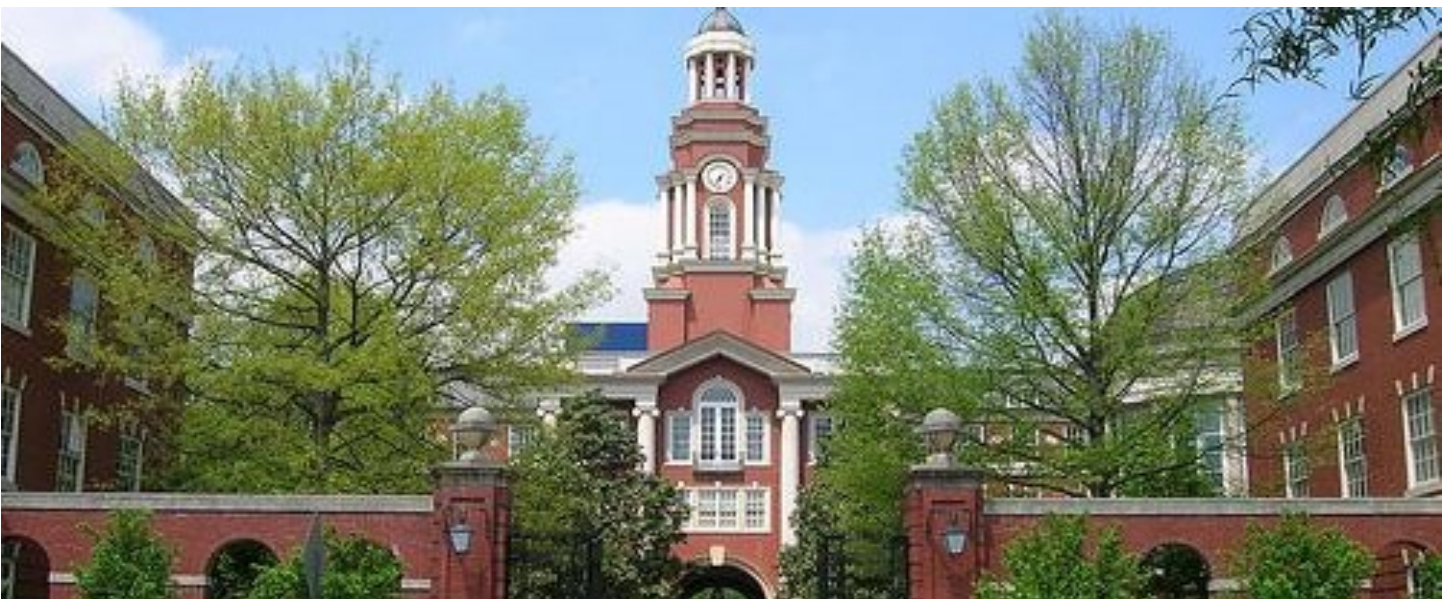
Howard Baker Jr. US Courthouse - Knoxville, TN
