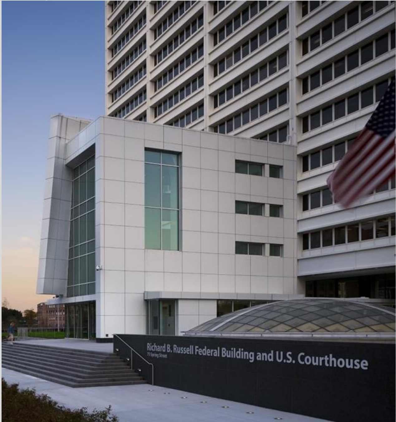
Richard B. Russell Federal Building and U.S. Courthouse, Atlanta, GA
