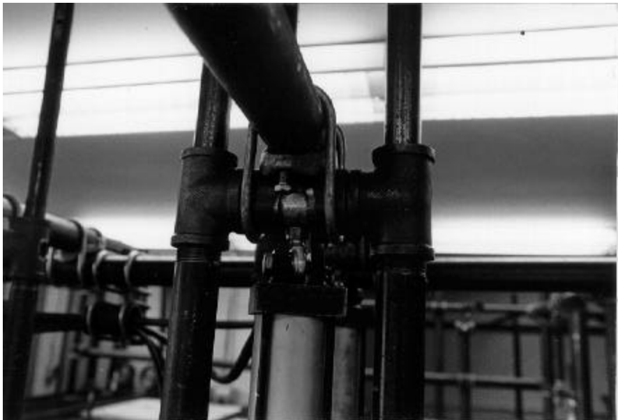
Figure 7c. The crossbar sleeve is rigidly attached to the main testing machine frame. The rod end fits through a slot cut through the sleeve and threads into a nut inside of the internal crossbar. The 1" access hole for the nut can be seen in the side of the Tee.
