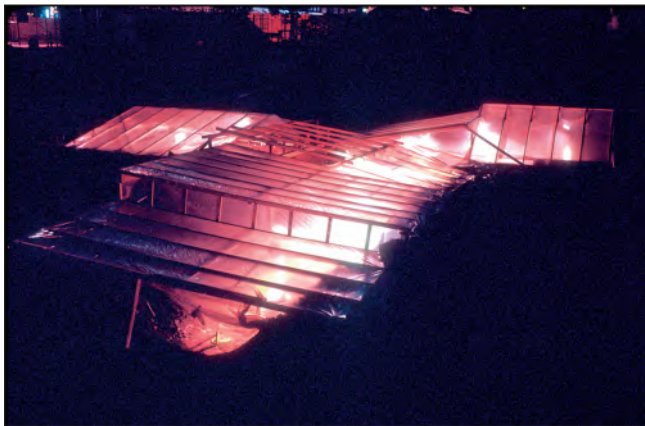
Figure 4. Excavation shelter erected to allow night and winter work (photograph by Dennis Seckler).
