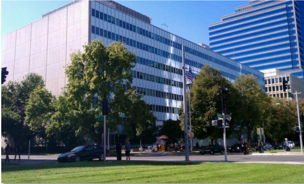
Figure 9: Photo of the exterior of the Moss Federal Building 5
