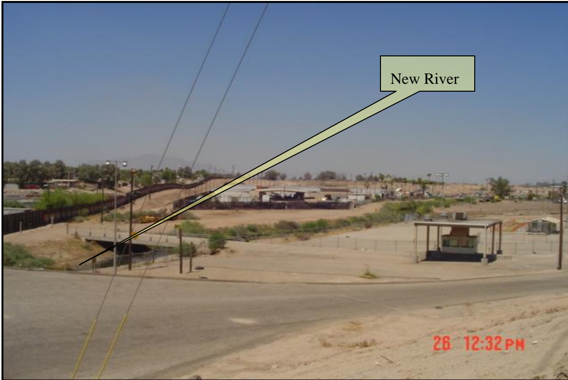
Figure 3.7-1. View looking west at the New River and vacated commercial inspection compound within the lower area of the site. Note the elevation difference from left to right.
