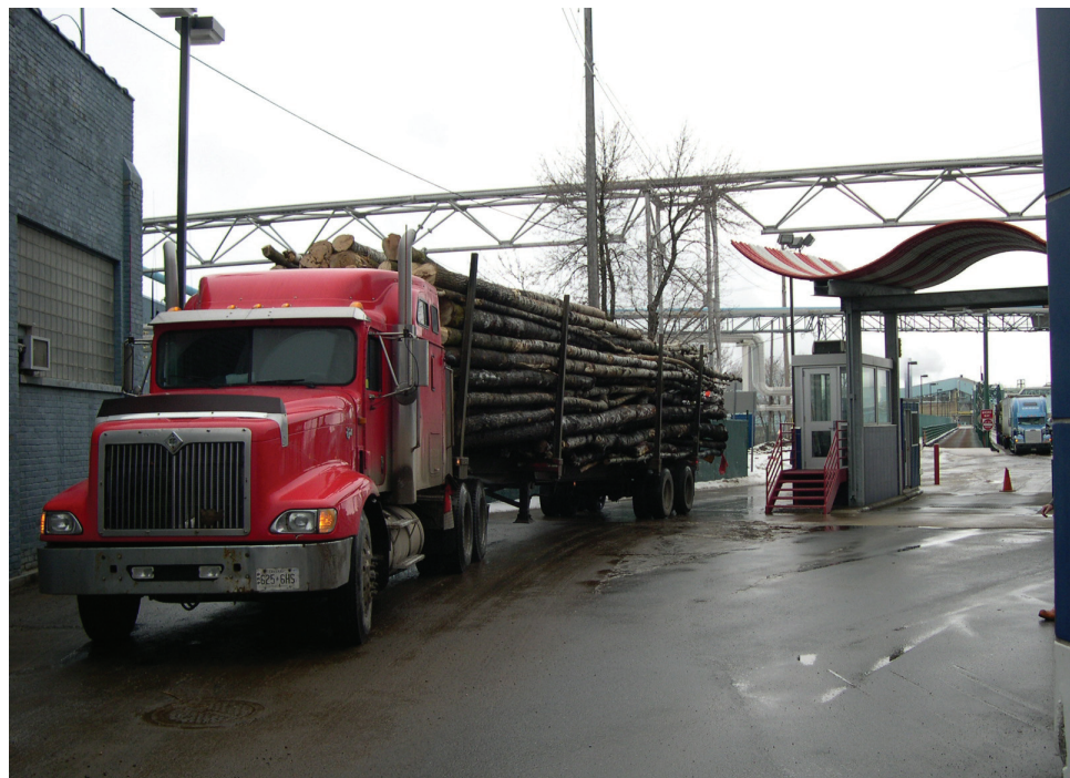
Deficiencies exist in the commercial vehicle inspection facility.
