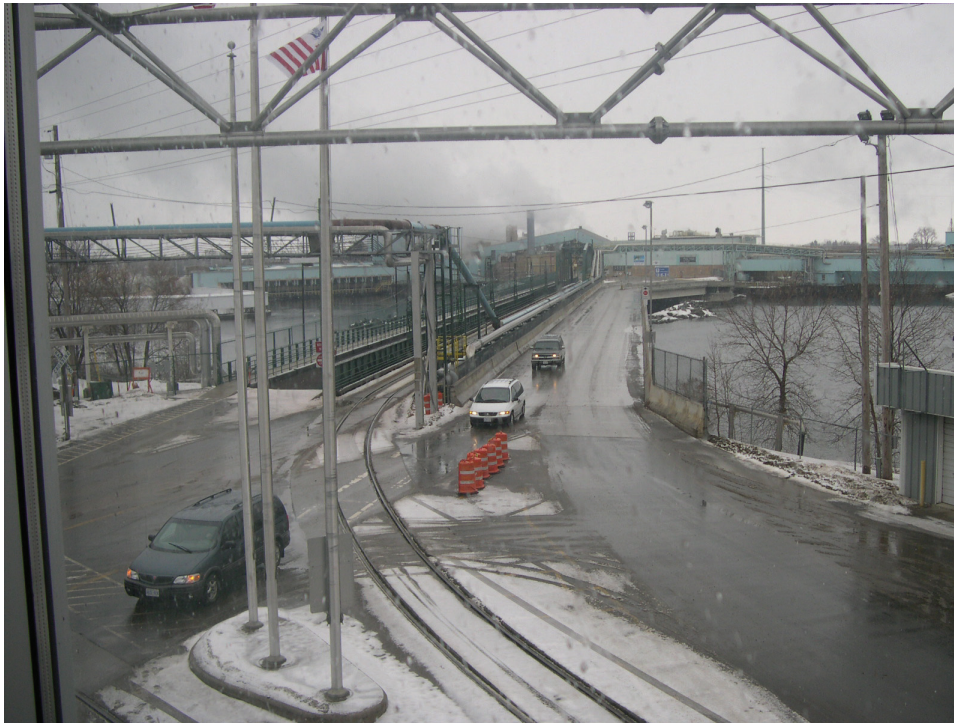
The MD&W Railway crossing the inspection lanes.
