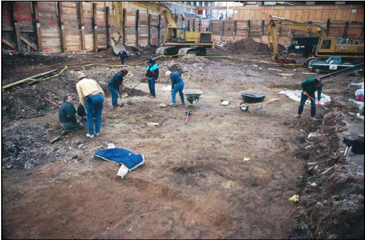
Figure 5. Cleaning interface between A and B horizons in the SE Area. View to the northeast.
