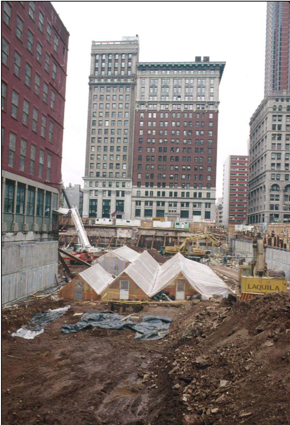
Figure 7. Excavation of a portion of the MID Area under shelters. View to the west.
