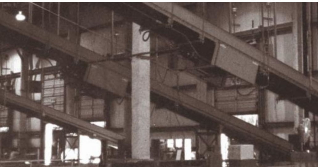
Conveyor Delivery System GSA/FSS, Palmetto, GA
