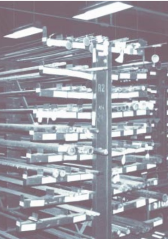
Steel Frame "C" Racks TVA, John Sevier Fossil Fuel Plant, Rogersville, TN
